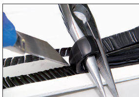
Pic 2: Peel of the aged bead using a plier
